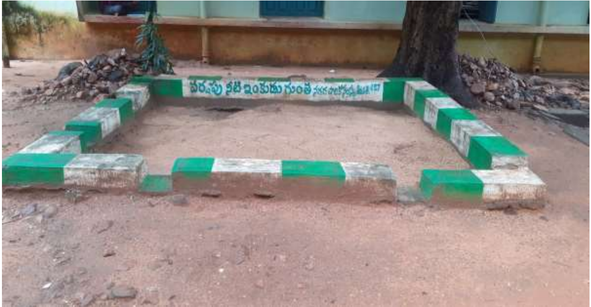
Rain water harvesting pit at western side of Electronics Dept
